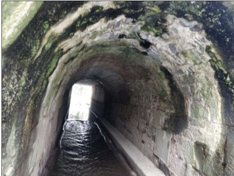
Plate 5.5 Lombardstown Bridge under the arch.
