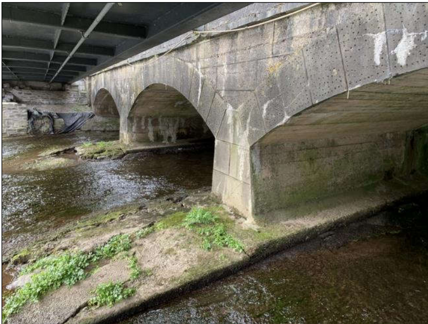
Plate 5.1 Killeagh River Bridge.
