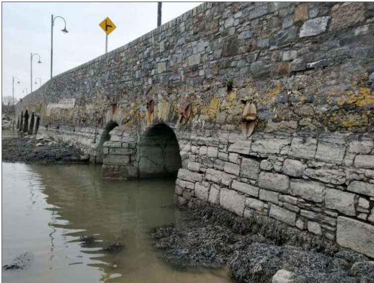
Plate 5.26 Blennerville Bridge Relief Arch.
