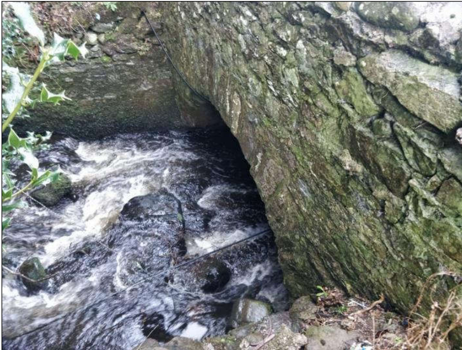
Plate 5.18 Glenbeigh National School Bridge.
