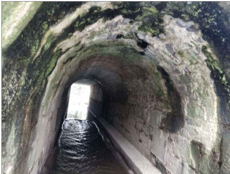
Plate 2.5 Lombardstown Bridge under the arch.
