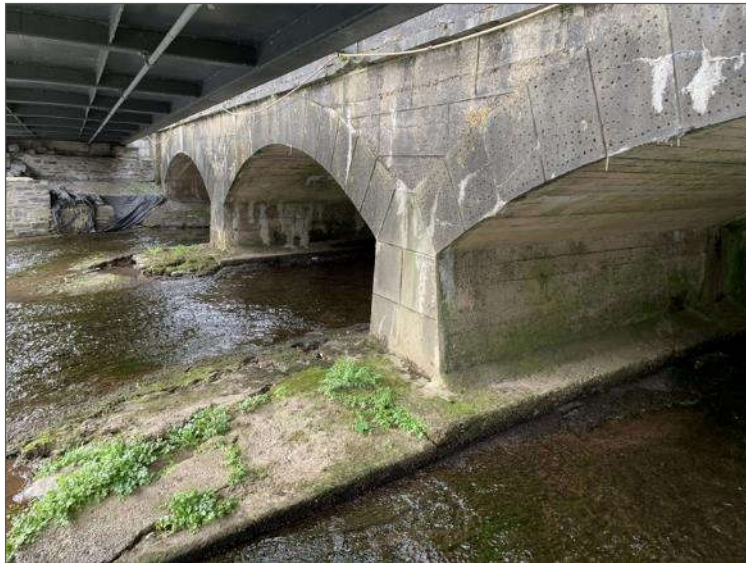
Plate 2.1 Killeagh River Bridge.
